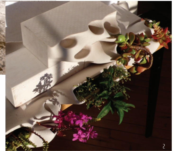
3D printed clay wall assembly
