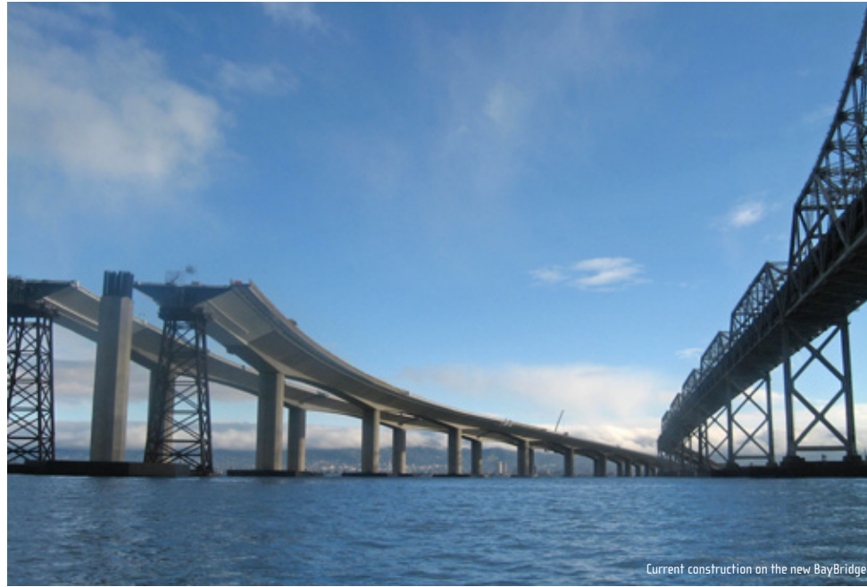
Current construction on the new Bay Bridge
